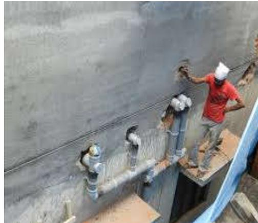
**Figure-4 Fixing of New Plumbing line**
