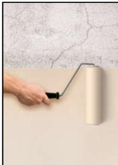
**Fig.7Crack Bridging coating**
