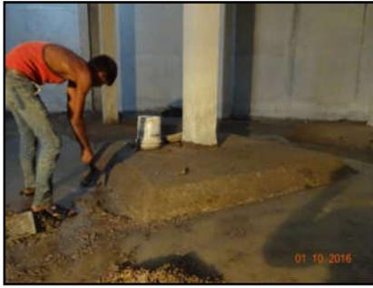
**Fig.8 Water proofing work inside the ESR**
